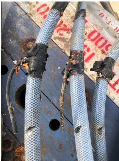
Figure 4 Wear on top-section mooring cables.
